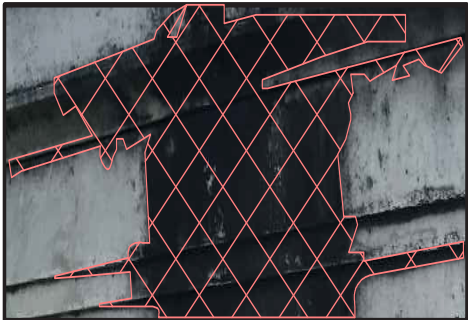
BIOLOGICAL GROWTH - grows when moisture is present and the substrate is not exposed to the sun
