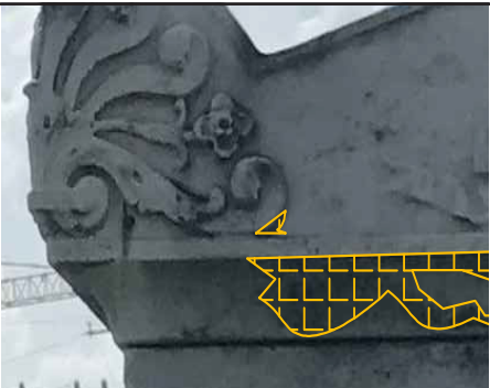
POLLUTION - staining due to airborne pollutants that leave a film over the surface of the substrate
