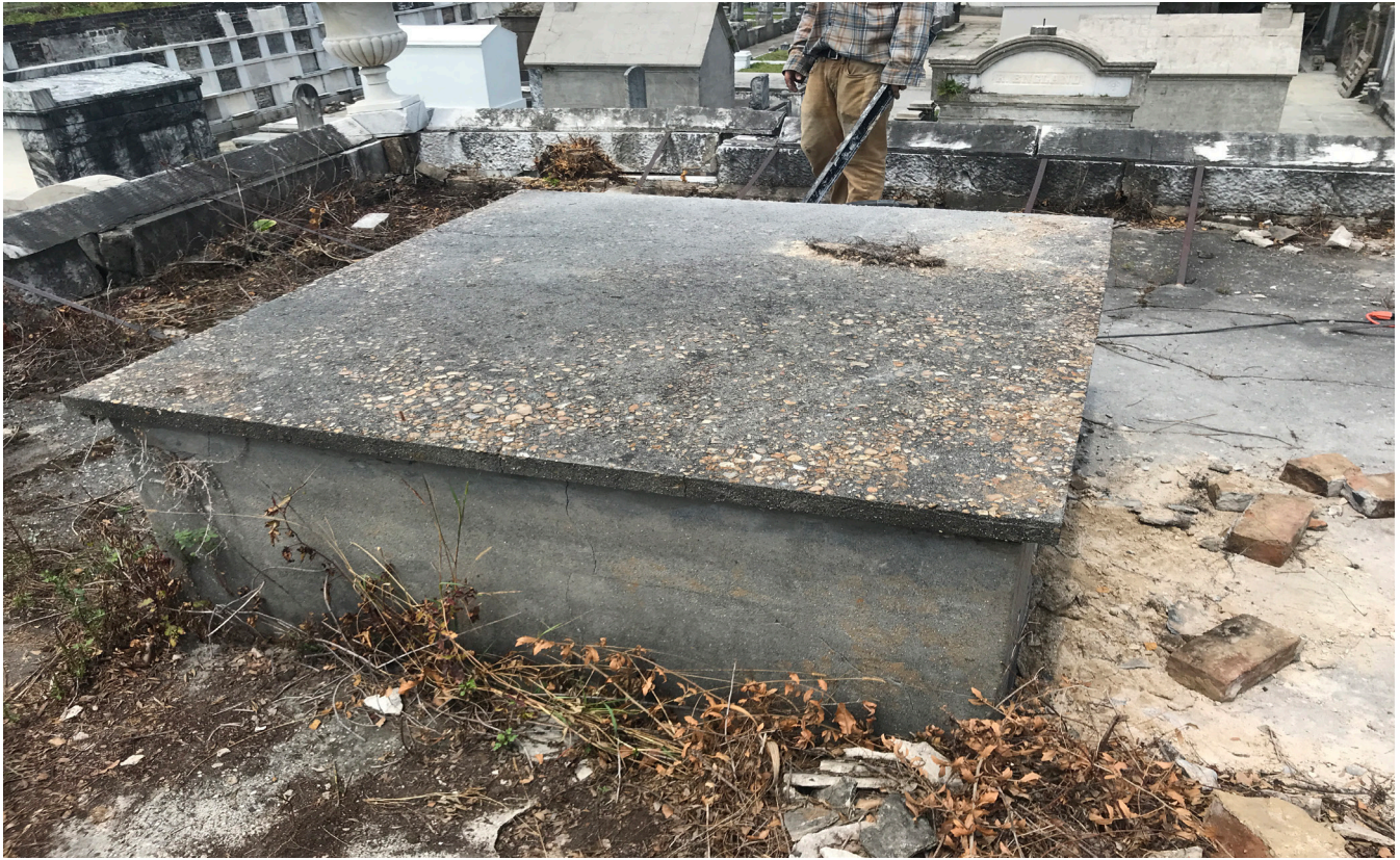
Figure 20. Photograph showing the raised portion of the roof of Teutonia Lodge.
