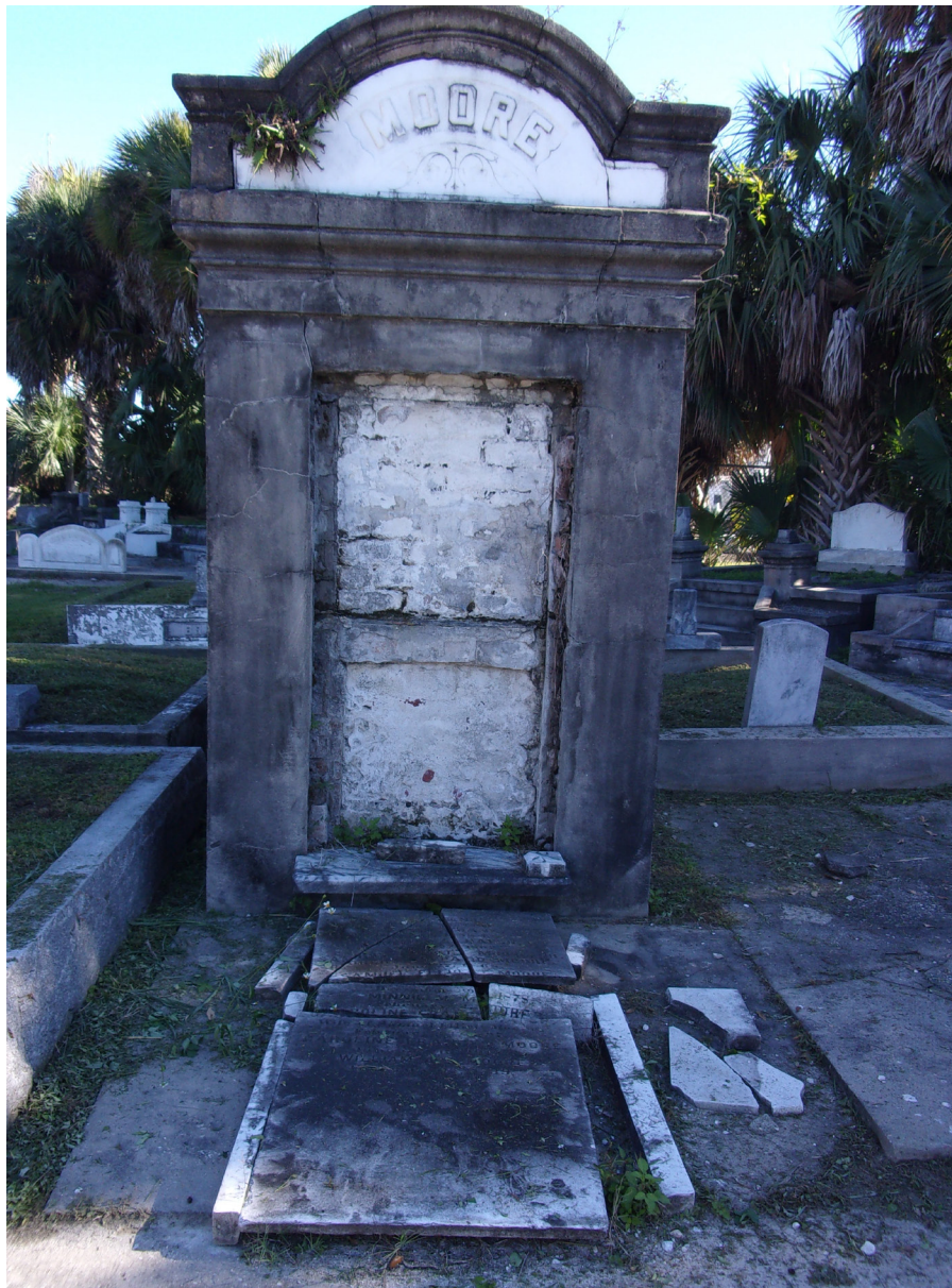
Figure 38. Tomb with fallen marble tablet, partially pieced together in front of the tomb.
