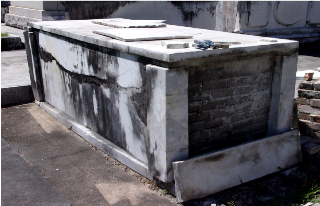
Figure 62. Platform tomb at OFR with a missing front tablet.
