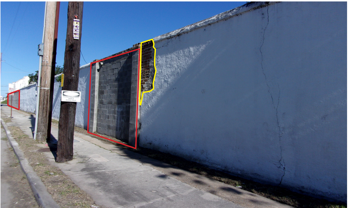
Figure 34. Photograph showing the repairs to the exterior Canal Street wall of OFR. Two cement sections are outlined in red, while the rest of the wall is constructed of brick covered in stucco, visible in the exposed patch outlined in yellow.
