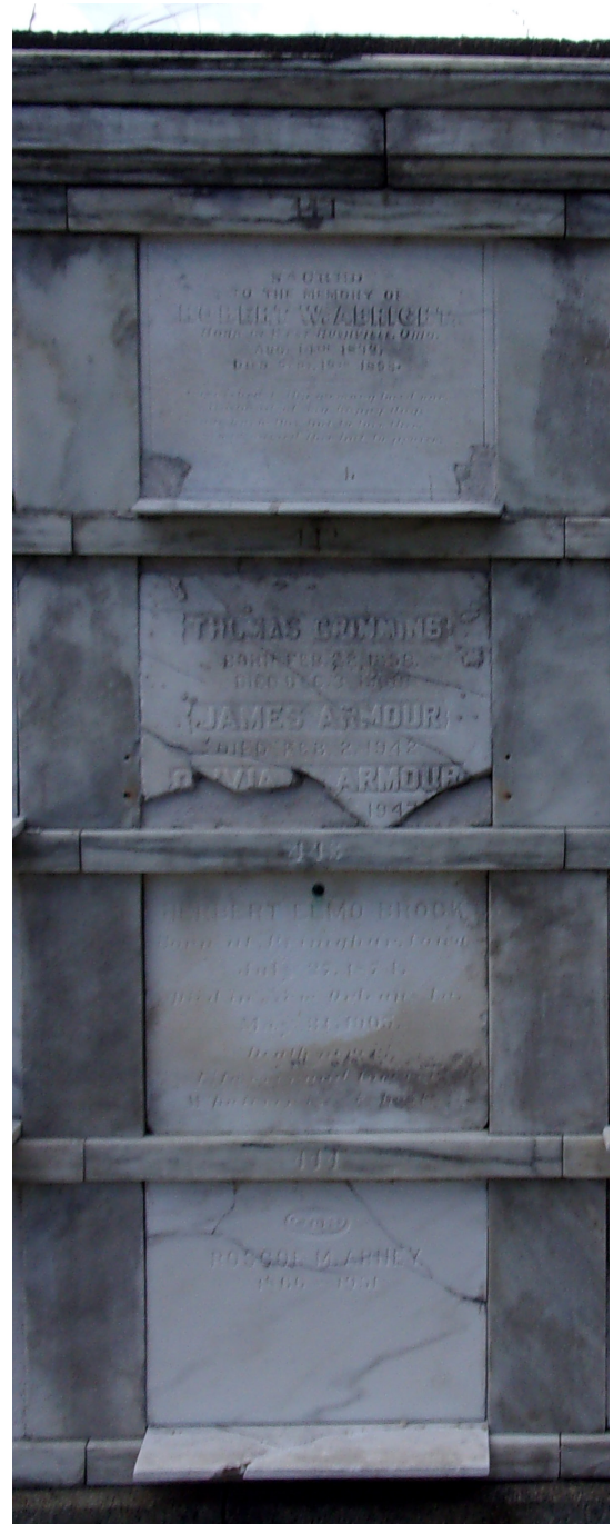
Figure 36. Repaired wall vaults 441 – 444, Southwestern wall.
