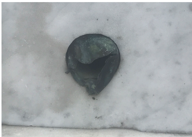
Figures 17 and 18. Copper pipes on the bottom corners of the northwest facade of Teutonia Lodge.
