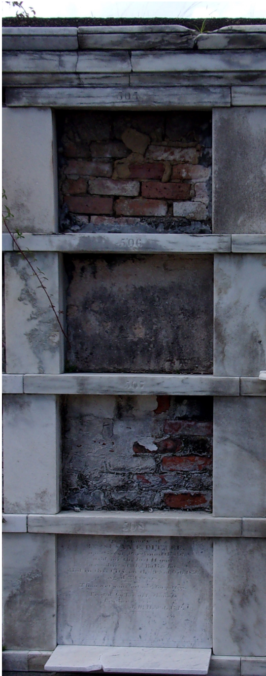
Figure 35. Wall vaults 505 – 508, Southwestern wall.
