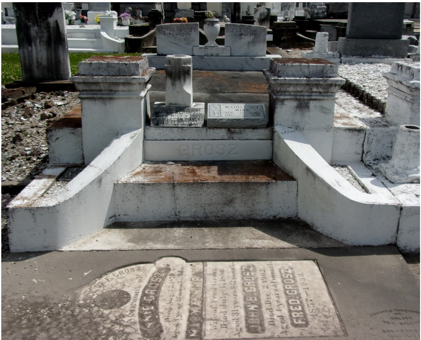
Figure 5. Grosz coping tomb, showing Rodehurst's intervention efforts. Taken by Emily Ford, 2012.
