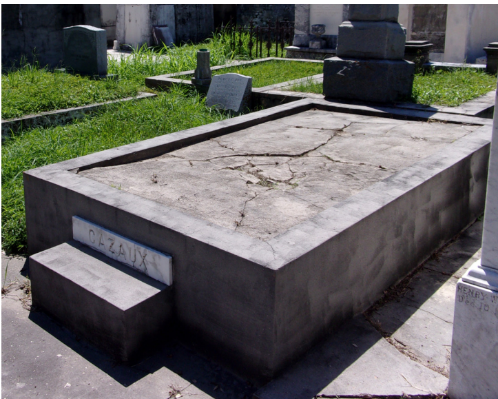
Figure 53. Coping grave in OFR that has been covered in cement due to rising remains.
