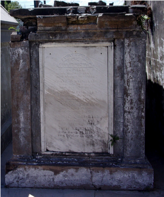
Figure 86. Significant missing material of the cornice and roof, cracking, spalling, and staining of front facade.
