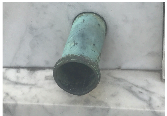
Figures 17 and 18. Copper pipes on the bottom corners of the northwest facade of Teutonia Lodge.
