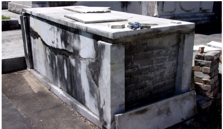
Figure 84. Two tombs in poor condition: significant vegetation growth and cracking. Missing bricks, stucco, and partially missing gate on the left.
