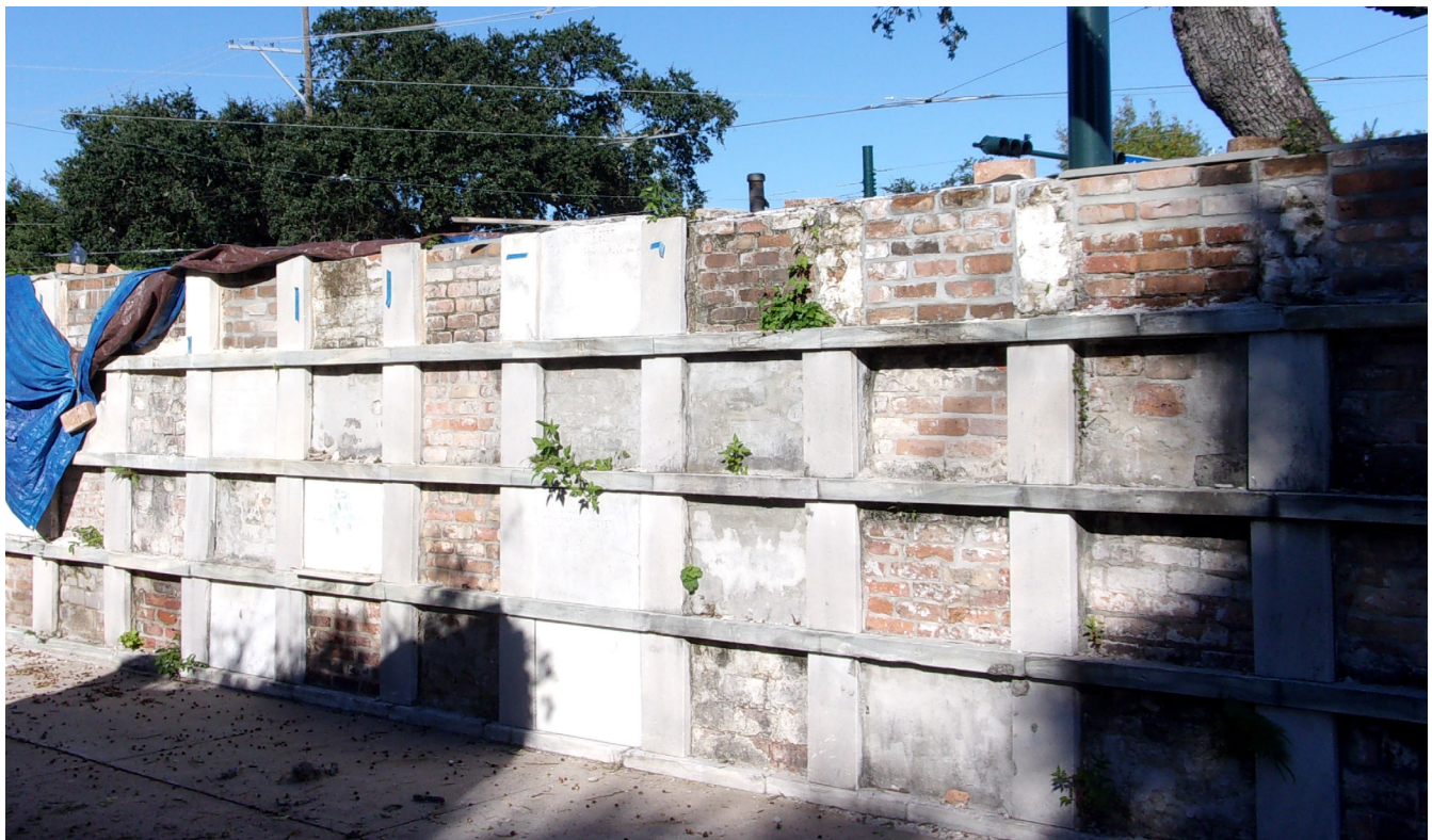
Figure 40. Photo showing the roof and cornice removed as work continues on the Northern (City Park Ave.) wall. The tarp (left-side of photo) is necessary in order to cover the open and vulnerable spaces of the roof.
