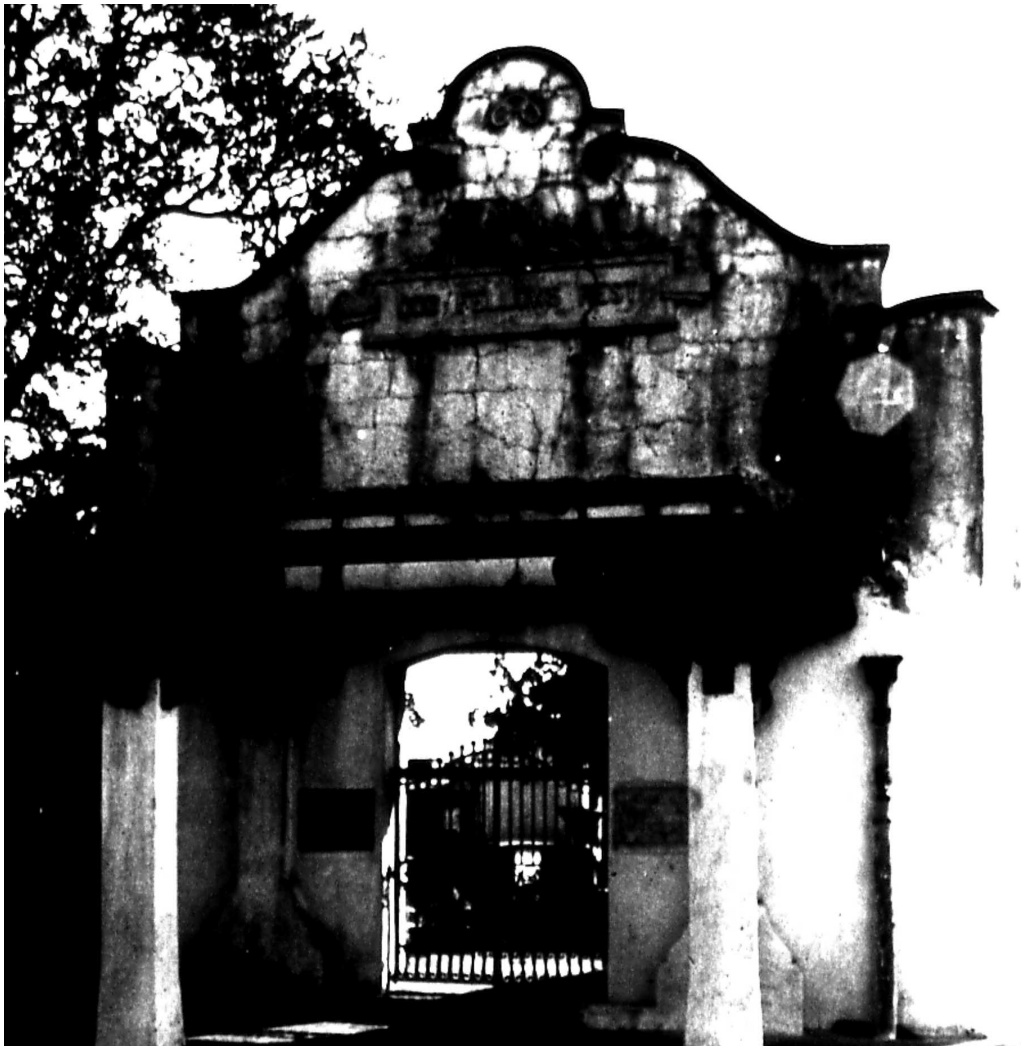
Figure 4. Entrance to OFR at the corner of Canal Street and City Park Avenue. Scan from 1980 Historic Cemetery Survey, Historic New Orleans Collection.
