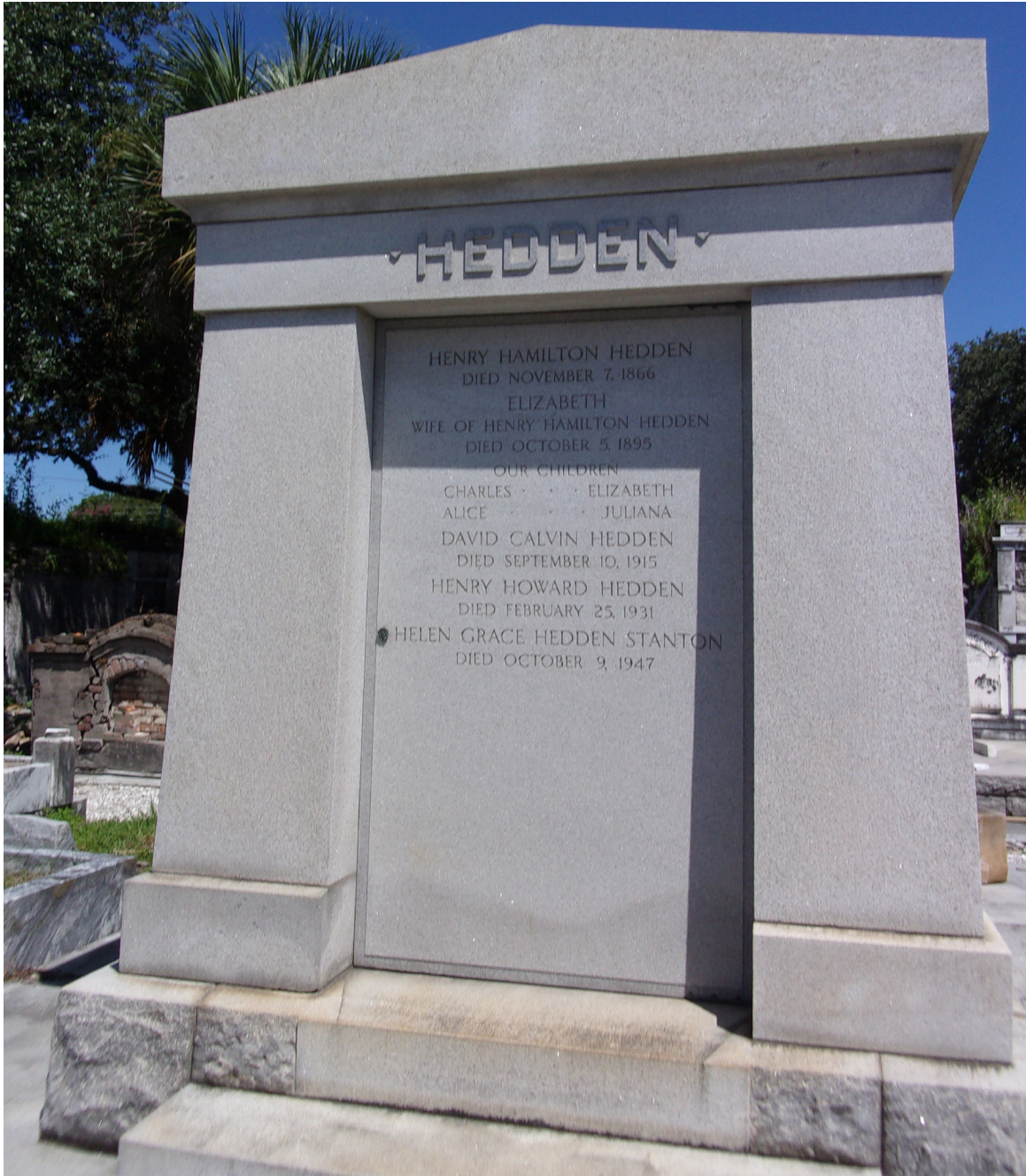
Figure 71. Large family tomb in good condition, but with some visible issues, such as the staining on the bottom steps.
