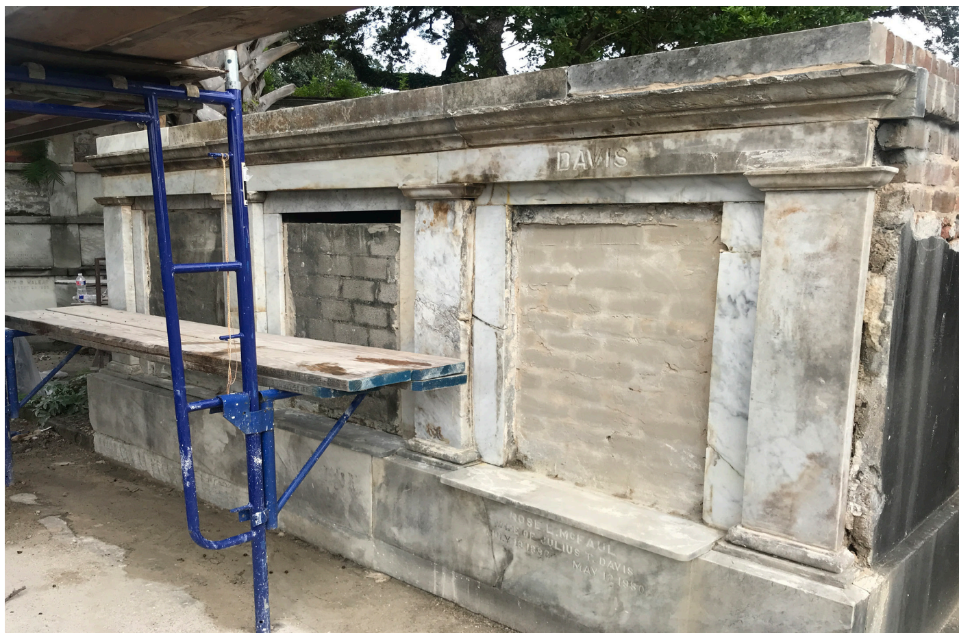
Figure 43. Newly reconstructed Davis tomb, still awaiting the installation of three front marble tablets, taken September 2018.
