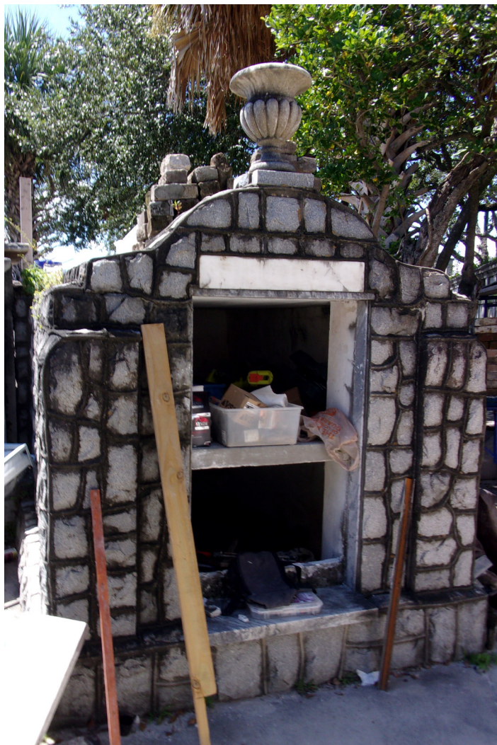
Figure 67. Tomb in Odd Fellows' Rest clad in granite rubble stone and thick Portland cement mortar joints. This granite rubble was most likely a twentieth century addition.
