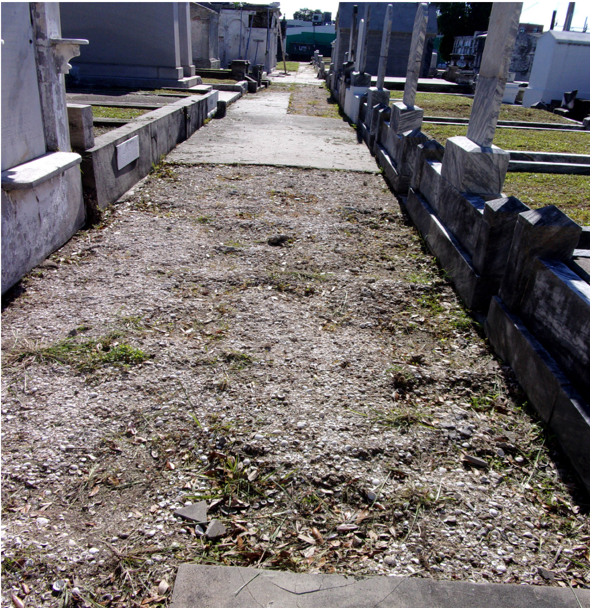
Figure 44. Partial removal of cement sidewalk. Eventually, all sidewalks will be removed and grass will be planted.
