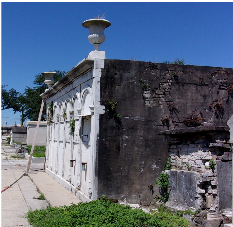
Figure 29. Teutonia Lodge. Rear corner, showing southwest and southeast facade. See Drawing A2, p. 22.
