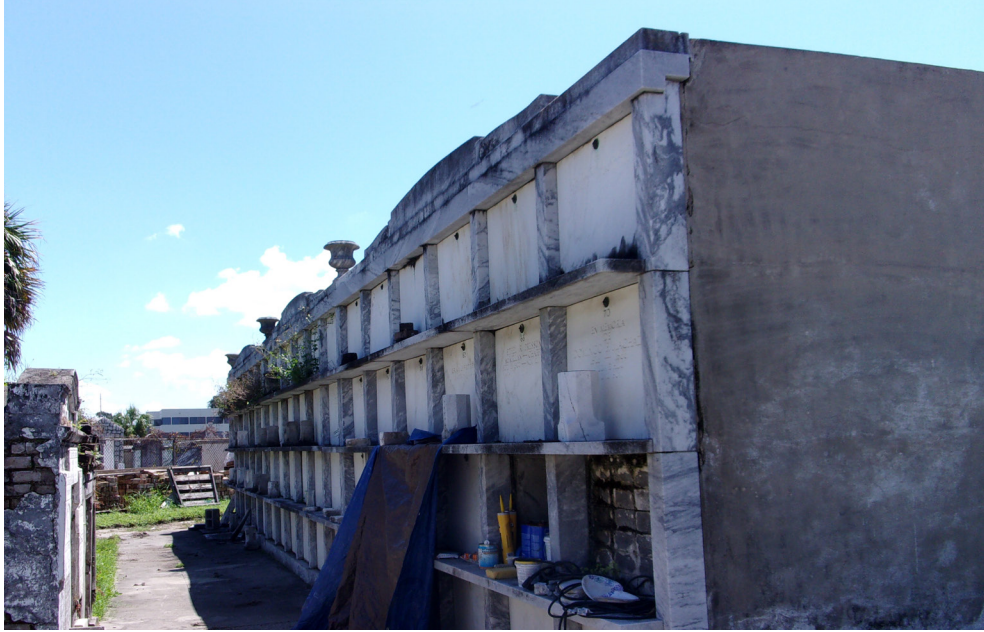
Figure 52. Block Wall Vault tomb.
