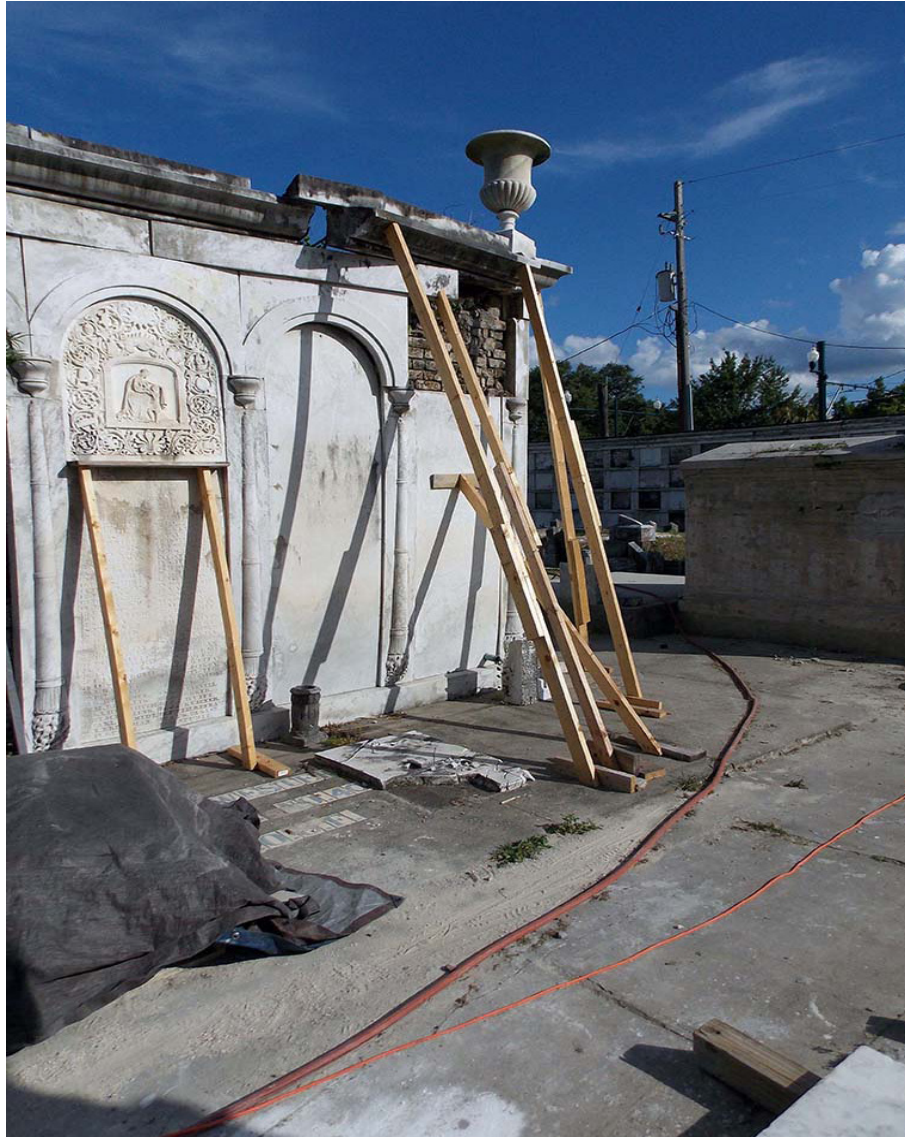
Figure 23. Southwestern facade after stabilization and partial removal of trees. Taken by Michael Duplantier, Sr., taken May 2018.
