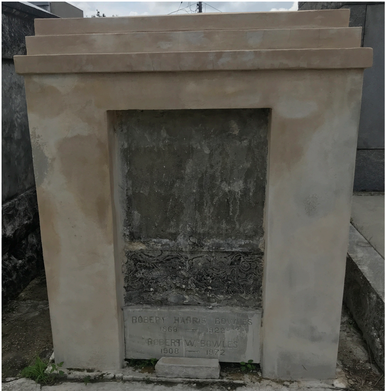
Figure 37. Repaired tomb with partially missing front tablet. Repaired in spring 2018.
