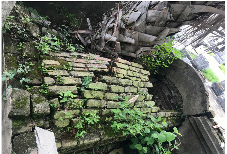
Figure 57. View from the rear corner of the barrel vault in OFR. Rounded roof and palm tree growing out of it are visible.
