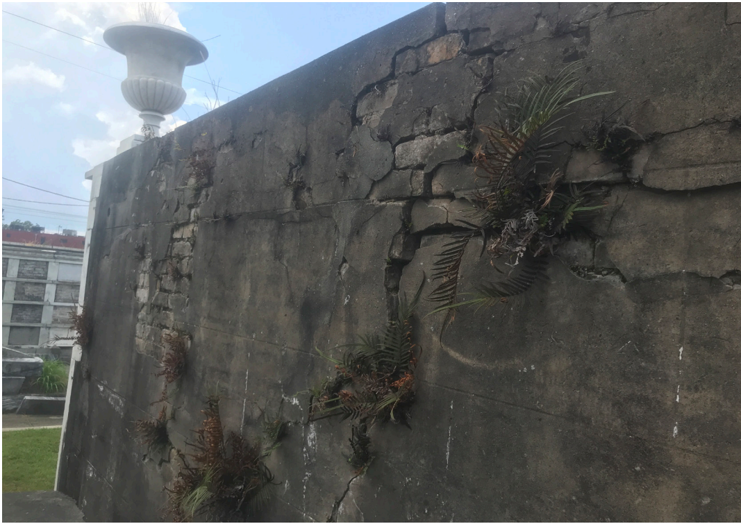
Figure 28. Teutonia Lodge. Southeastern Facade.
