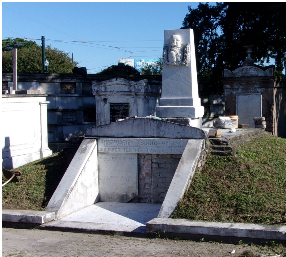
Figure 74. This tomb is not as exposed to the elements due to it being a tumulus, helping to contribute to its maintained condition. It has minor staining and has recently been cleaned.
