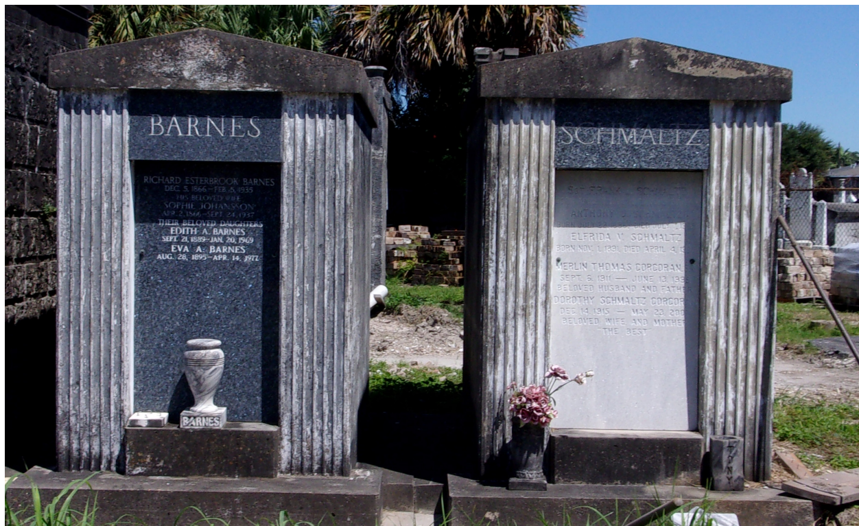
Figure 76. Two structurally sound tombs with some spalling. Cleaning is needed.
