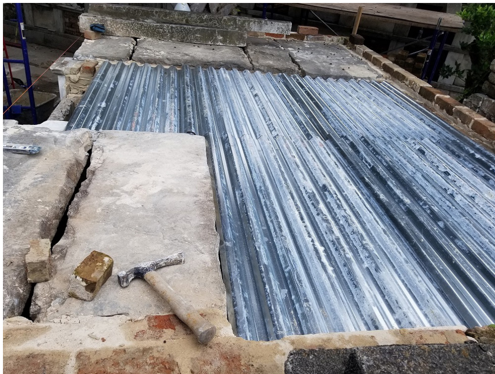
Figure 42. New corrugated steel roof, as a part of the Davis tomb reconstruction, taken by Michael Duplantier.
