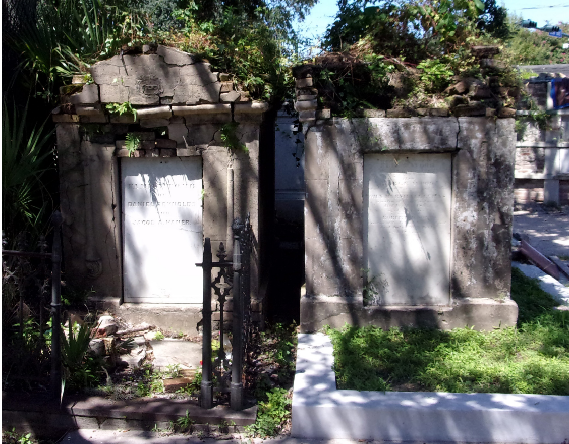
Figure 84. Two tombs in poor condition: significant vegetation growth and cracking. Missing bricks, stucco, and partially missing gate on the left.
