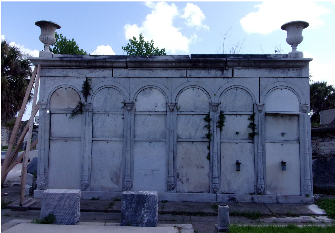
Figure 11. Southwestern facade of Teutonia Lodge, taken by the author, July 2018.
