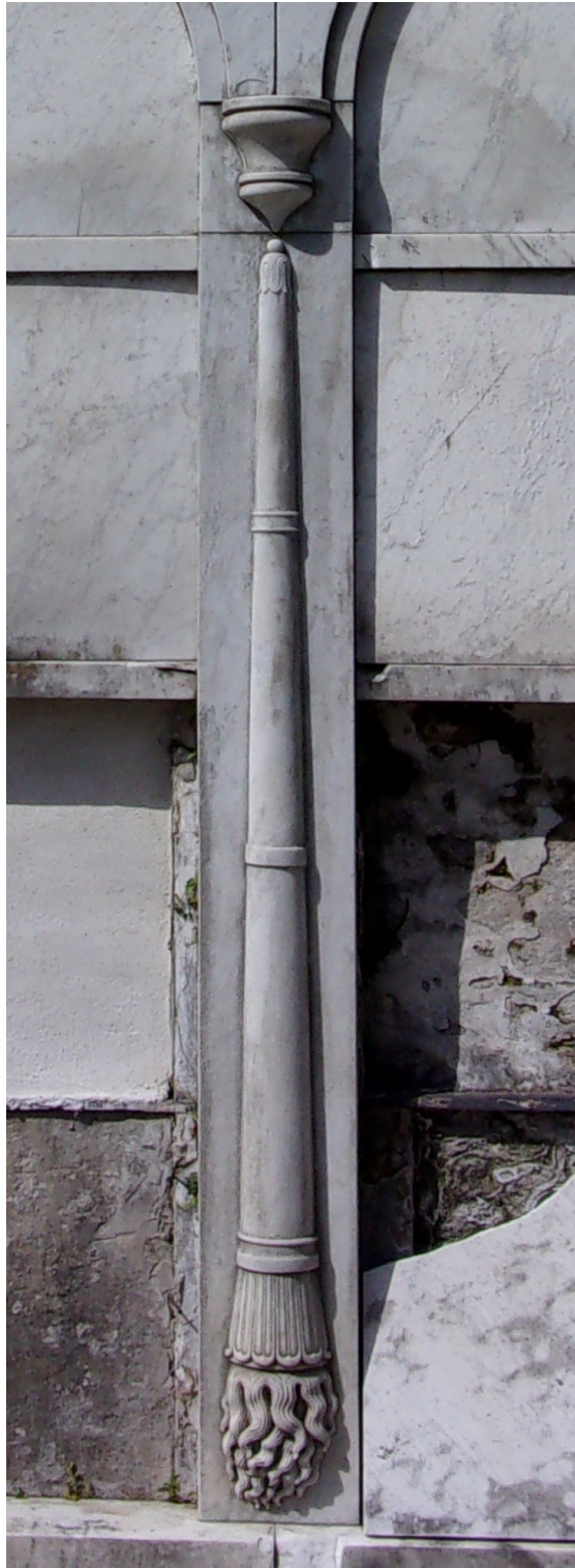
Figure 31. Teutonia Lodge. Inverted torch detail located on the three primary facades. See Drawing B2, p. 24.
